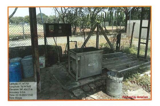
The maintenance department in the campus collects approximately 800 kilograms of food waste from hostels every day that is converted into biogas by processing through the biogas plant available in the campus. 19 kilograms are produced everyday that saves the consumption of commercial cylinder.
